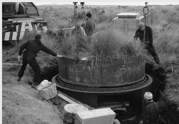
Figure 3.5 Large weighing lysimeter at Glendhu being installed. The weighing mechanism can be seen underneath.
