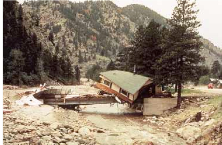
Figure 14–27 The 1976 Big Thompson Canyon flood in Colorado lifted this house from its foundation and carried it downstream. (USGS)
