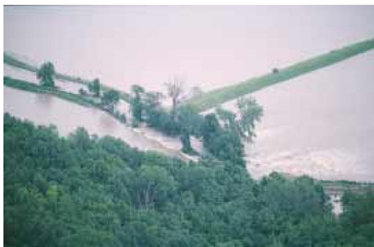
Figure 14–29 Flood waters pouring from the channel of the Missouri River through a broken levee onto the flood plain in Boone County, Missouri. (Stephen Levin)
