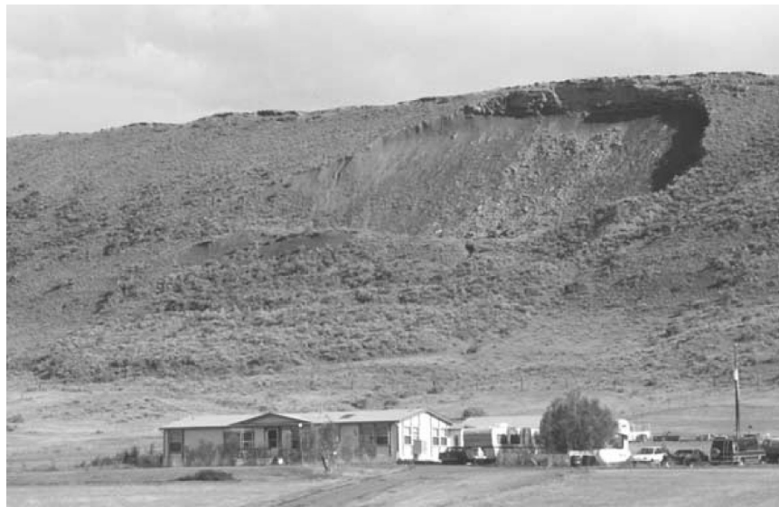
Plate 3.1 Shallow rotational landslide, Rockies foothills, Wyoming, USA. (Photograph by Tony Waltham Geophotos)
