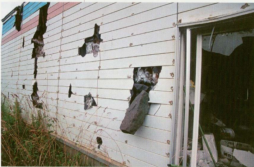
▲ Fig. 13.12. Blocks ballistically emplaced into wall of Kindergarten building during 2000 eruption of Usu volcano (Hokkaido, Japan). Distance to crater about 1 km
