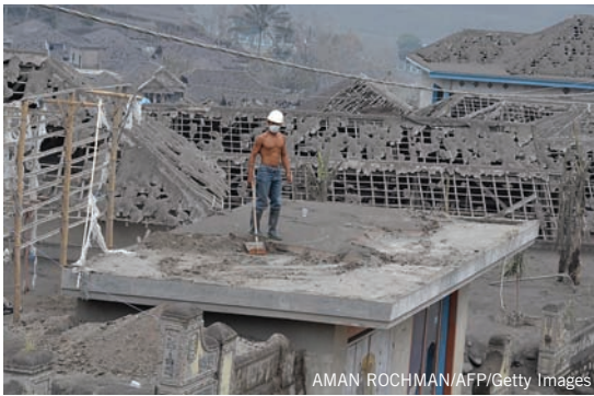
Ash and other pyroclastic materials can collapse roofs, or completely cover buildings.
