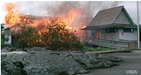
Lava flows can destroy homes, roads, and other structures in their paths.
