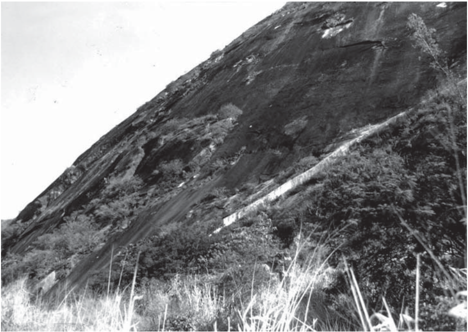
FIGURE 1.16 Exfoliation loosening granite slabs. Impact wall on right was constructed to deflect falling and sliding blocks from buildings on lower slopes. Damage from falls and slab slides is a serious problem in Rio de Janeiro.
