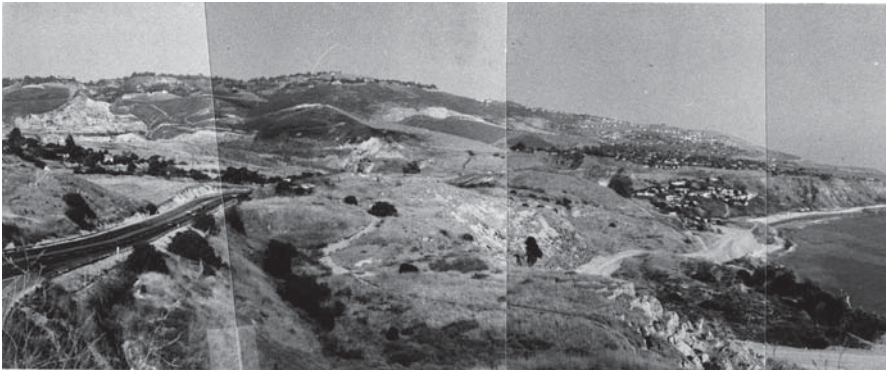
FIGURE 1.38 Panorama of the Portuguese Bend landslide looking south. The highway on the left is continually moving, and the old abandoned road appears in the photo center. The broken ground on the right is the head scarp of rotational slides in the frontal lobe of the unstable mass (photo taken in 1973).
