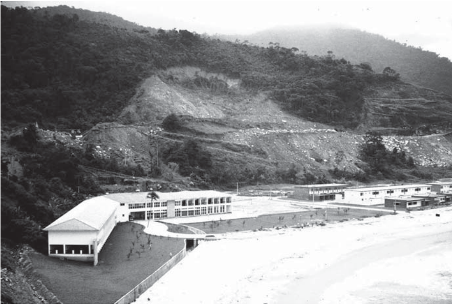
FIGURE 1.90 Debris avalanche scar along the Rio-Santos Highway at Praia Brava, Itaorna, Brazil. The slope form was concave; location is around the bend from Figure 1.89.
