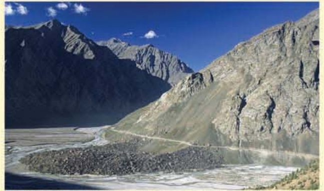
Road across scree and debris of large landslide, Indian Himalaya.
