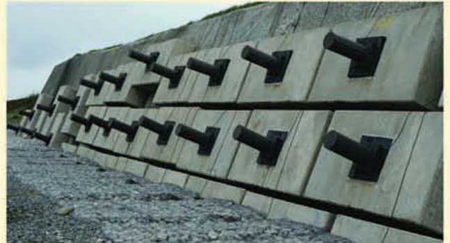
Ground anchors supporting landslide at Hoar Edge, Pennines.
