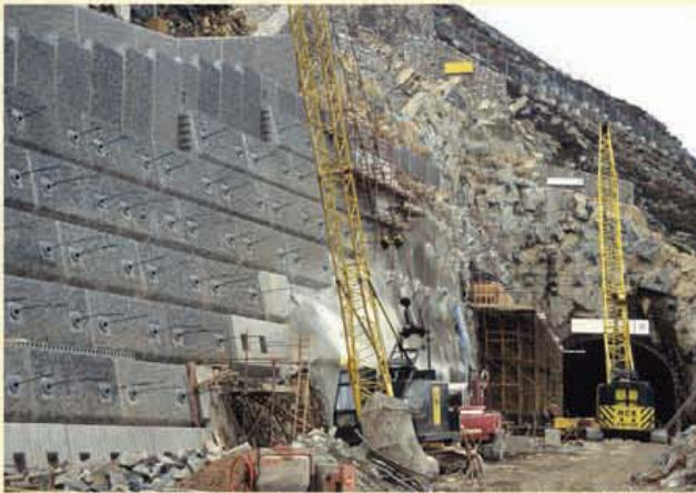
Anchored panel wall retaining poor rock at tunnel portal, Wales.
