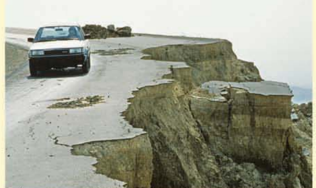
Failure of steep hillside after unusually heavy rain, Jordan.
