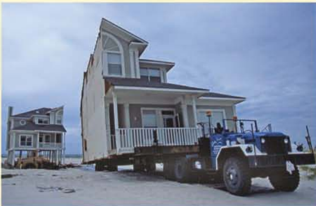
Moving houses threatened by erosion and beach loss, Alabama.
