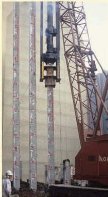
Driven piles in alluvial sand, England.
