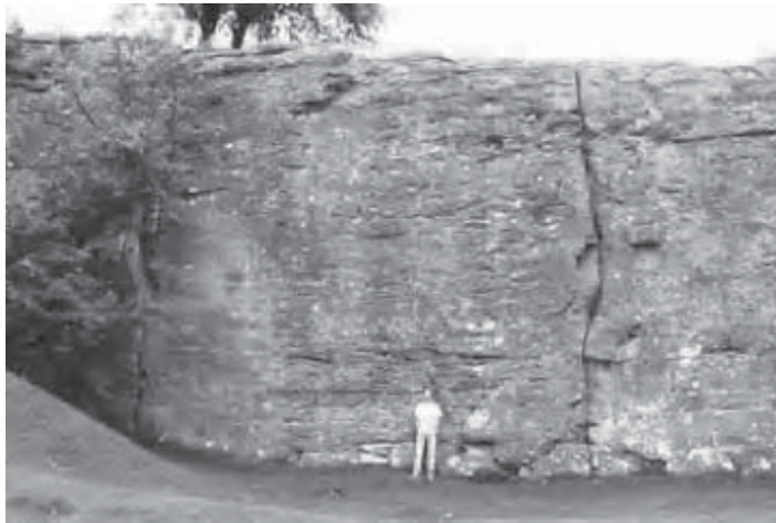
Figure B4-4.3 More distant view of Brockram at Hoff's Quarry. Note the fully persistent, near-vertical master joints about 40m apart, which will control mass permeability. Evidently joints from this set would only be intersected using inclined rather than vertical boreholes.
