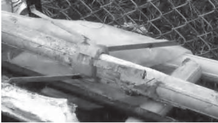
Figure 4.44 Exhumed inclinometer tubing. Four grooves inside (ridges outside) are guides for the wheels on the inclinometer instrument. The device with arms is a spider, which becomes fixed in position against the walls of a borehole whilst the tube can pass up or down inside. It is magnetic and a probe down hole can locate it and measurements can be made of settlement (as well as inclination).
