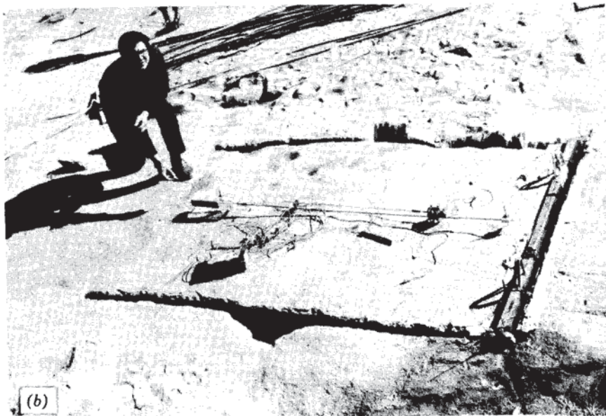
Figure 3.22 Large uniaxial compression tests conducted in-situ by TerraTek on Cedar City Quartz Diorite. (a) Drilling a line of 1-1/2-inch diameter holes plunging 60° to create an inclined slot forming one side of the triangular prism “specimen.” (b) A view of the test site showing flat jacks at one end and extensometers for relative displacement measurement during loading. (Courtesy of H. Pratt.)
