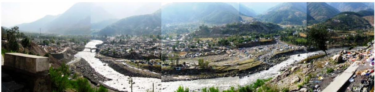
Fig. 6 Panoramic photo of the destroyed city of Balakot
