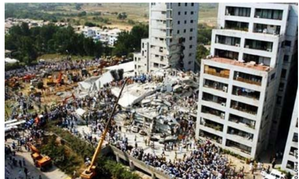
Fig. 10 Margala Tower collapse in Islamabad (Associated Press, Oct. 2005)
