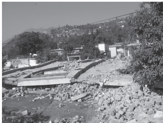
▲ Figure 25. Out-of-plane failure (Muz).
