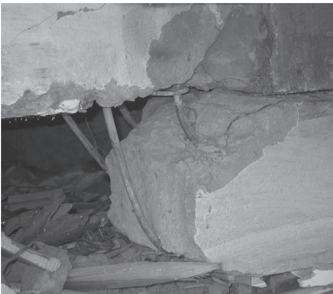
▲ Figure 16. Smooth reinforcing steel bars (Blk).
