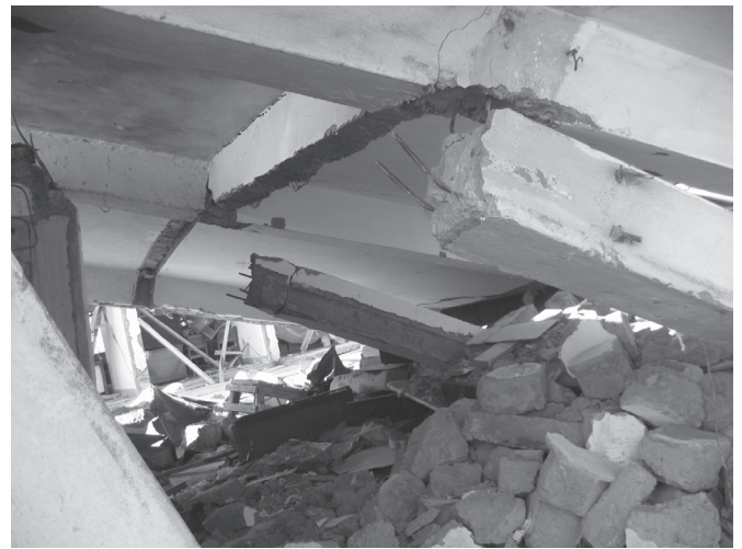
▲ Figure 13. Anchorage and development length (Blk).
