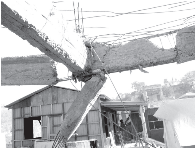
▲ Figure 12. Strong beam–weak column (Blk).
