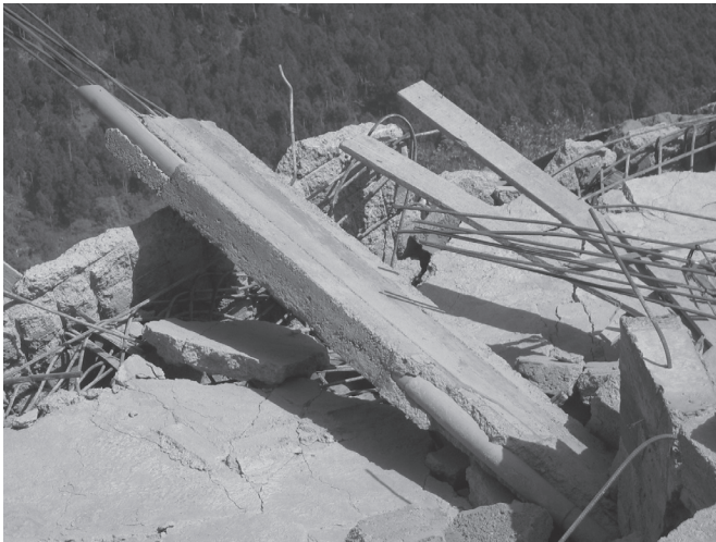
▲ Figure 18. Construction practices (Blk).
