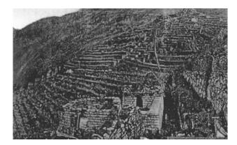
**Figure 6.** Machu Picchu Agricultural Terraces (by Hiram Bingham in 1912) showing tons of undamaged walls made by stone which resisted Llndslides and earthquakes. Drainage systems (surface and subsurface) were built to manage average annual rainfall of 1940 mm [69].
