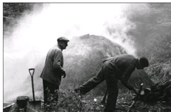
Figure 8.3 Operation of a mound kiln showing the heavy smoke emitted during the carbonization process
